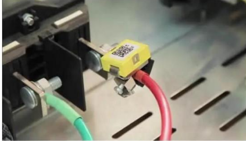
● Installed on Cable Joint of GCK Drawer
