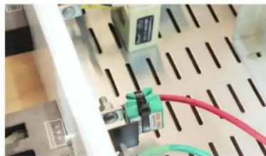
● Installed on Cable Joint of GCK Drawer
